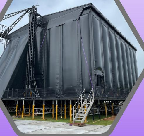
**Unmatched Roof Weight Capacity at 55 Tonnes with each PA Side Rated to 15 Tonnes.**
